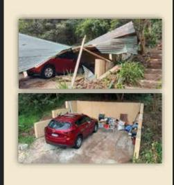
Make Safe Project Re-fixing the torn off roofing.
